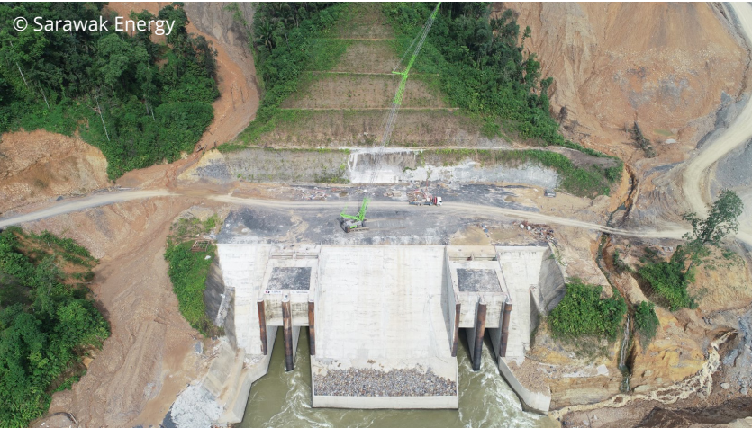
Work in progress at Baleh Dam site where a diversion tunnel is being built.
